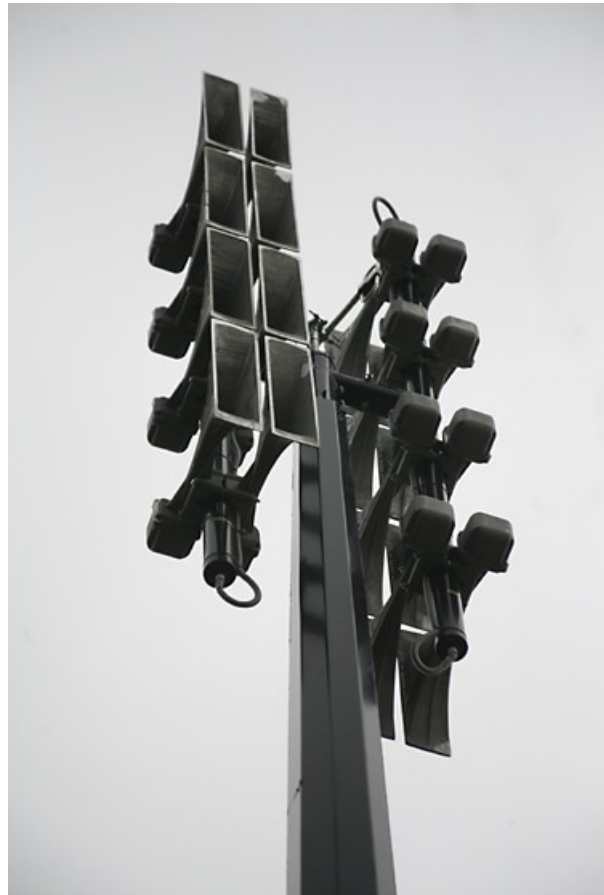
Mt Nebo Emergency Warning System
